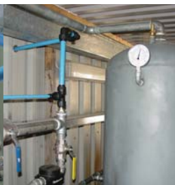
5. System complete in 2 days
